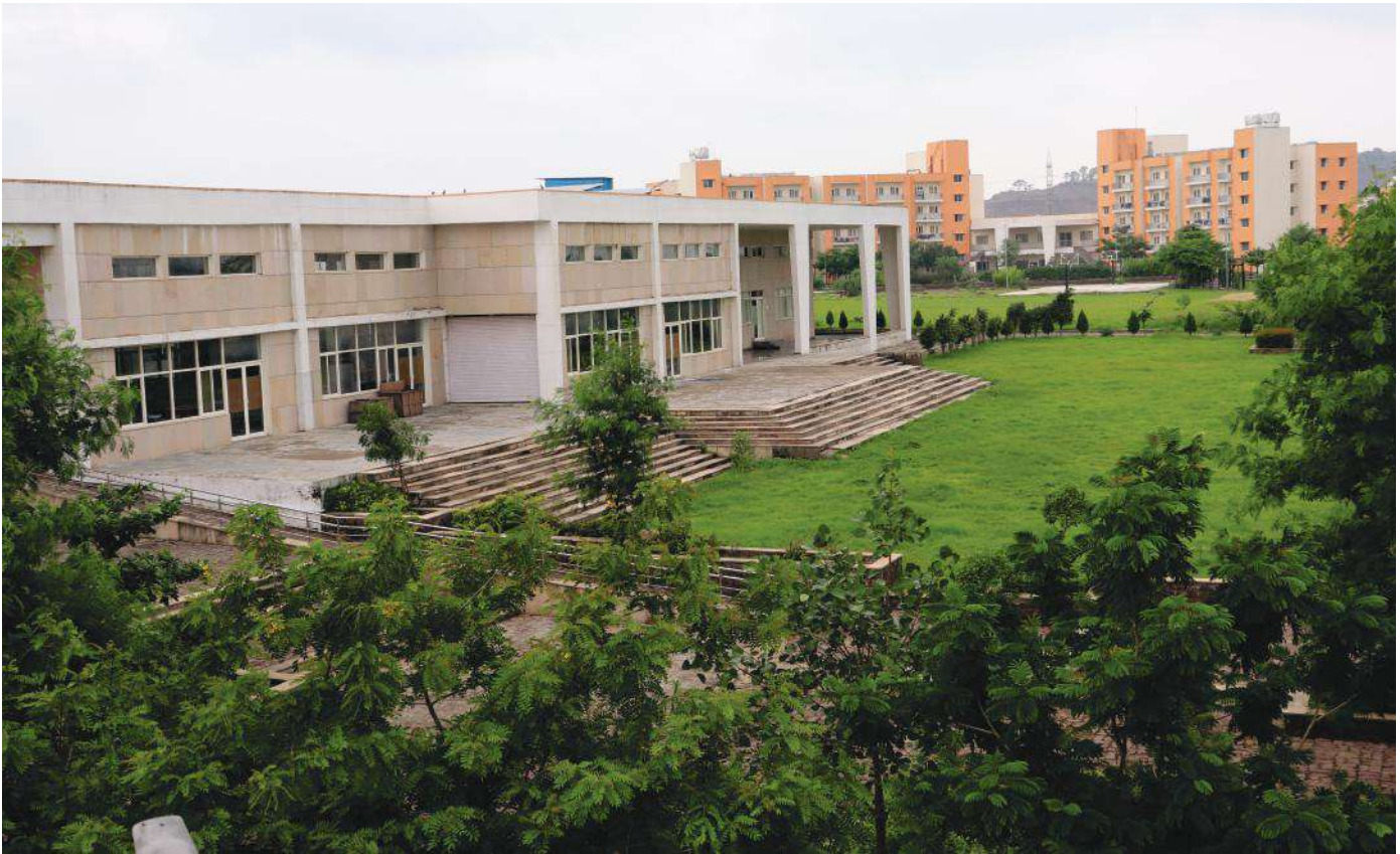
National Institute of Design, Madhya Pradesh campus
